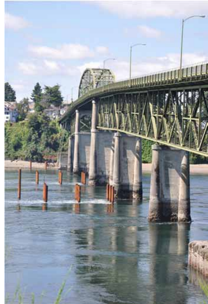
SR 303 - Manette Bridge (1920)
