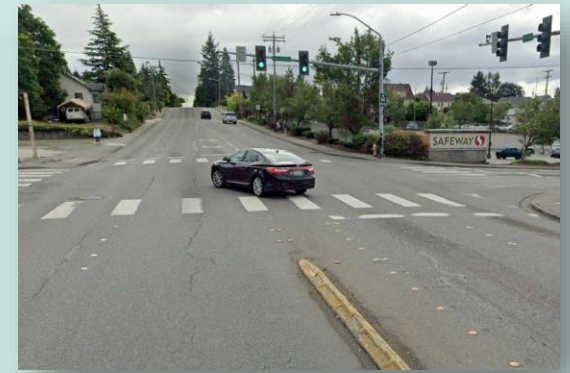
11 th at Callow Lacking Left-Turn Lane (Numerous Documented Rear End Collisions)
